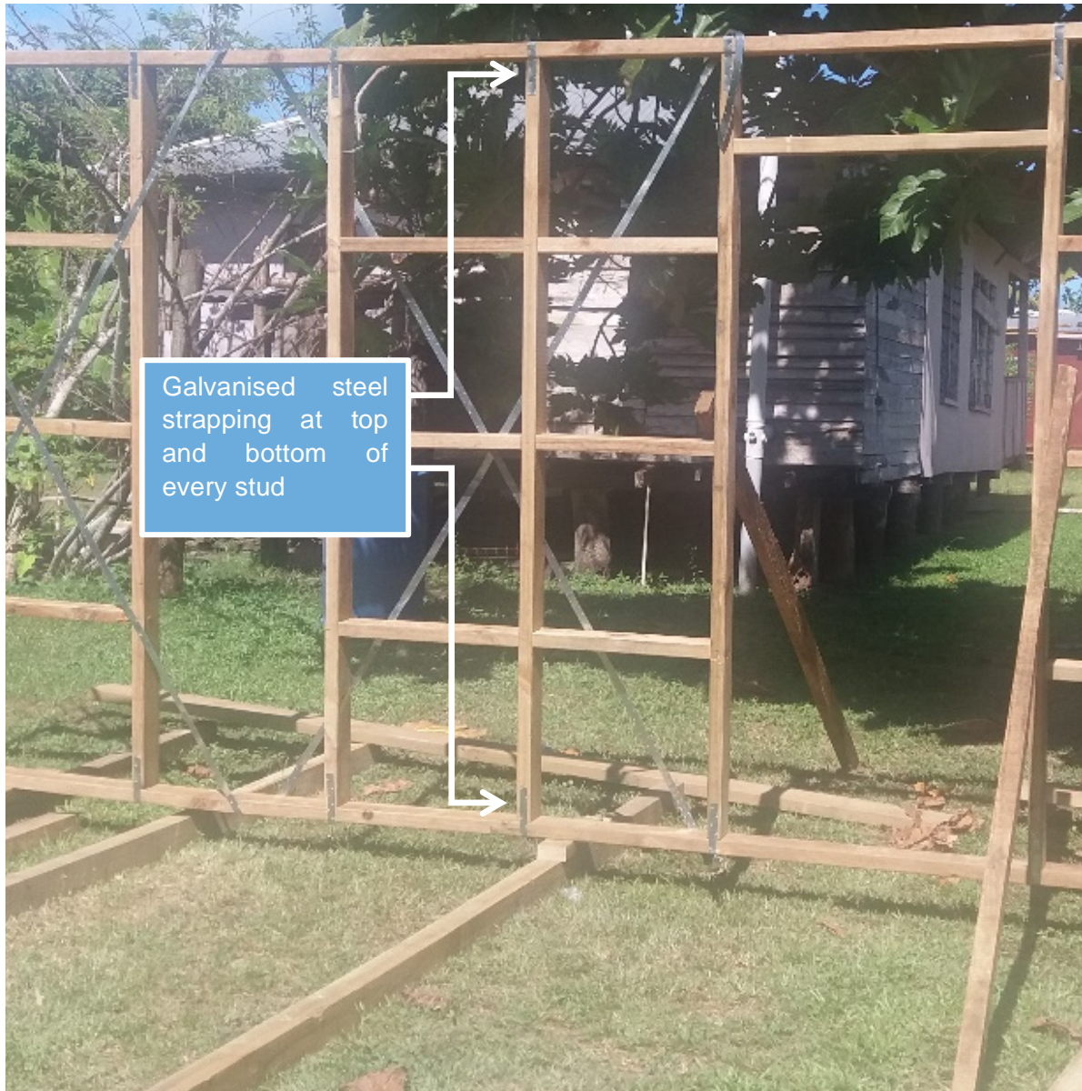
Figure A14: Stud wall frame with galvanised steel cyclone strapping (Source: Fiji Rural Housing Unit)
