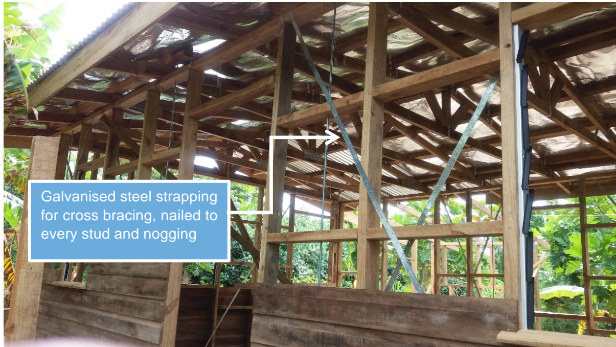
Figure A16: Stud frame wall with galvanised steel strap bracing (Source: Fiji Rural Housing Unit)
